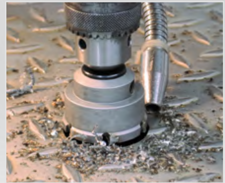
Drilling in checker sheet
