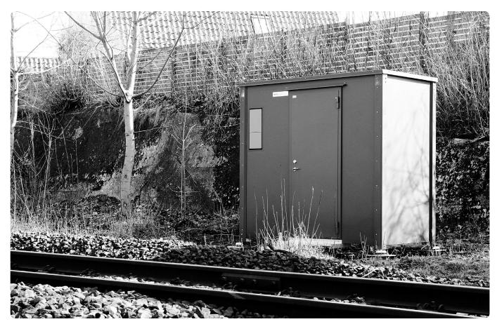
The walls, roof and floor are sandwich laminated building elements with a light frame construction inside - which for example could be an aluminum frame. Inside the shelter the walls can be delivered with different kinds of material. The most common version is with birch plywood, which gives the user an easy installation of the equipment.
